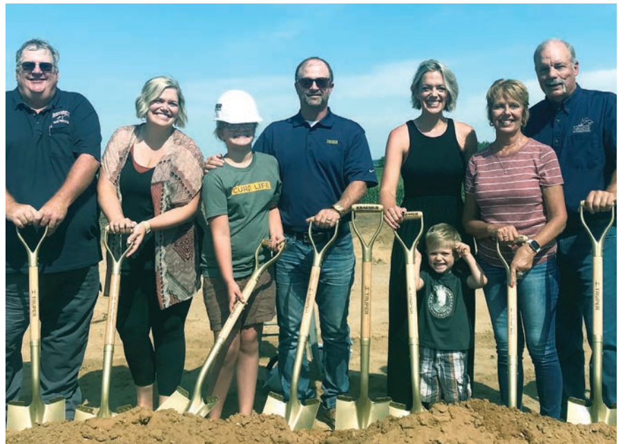
Decatur Dairy broke ground this week on a major expansion to the existing cheese plant. In the photo above (left to right) are: Steve Carpenter, president of Decatur Swiss Cheese Cooperative, Sierra Stettler, Decatur Dairy, Sutton Guilbault, Aaron Guilbault, Decatur Dairy, Shaya Guilbault, Decatur Dairy, Shaw Guilbault, and owners Glennette (George) Stettler and Steve Stettler.
